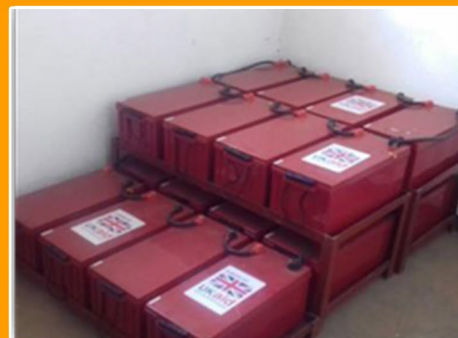
9KWP Three phase solar backup system for cooling milk. Mapuyu Milk Bulking Group- Chileka-Lilongwe
