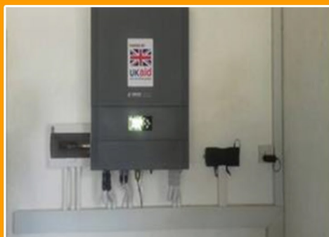
9KWP Three phase solar backup system for cooling milk. Mapuyu Milk Bulking Group- Chileka-Lilongwe
