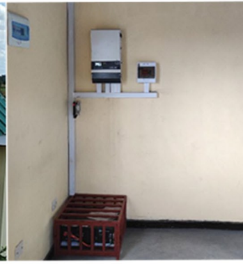
Off-grid Solar System for Village Clinic in Mchinji. 1.1Kw of Solar Inverter and 2.4kwh 24 V Lithium Battery
