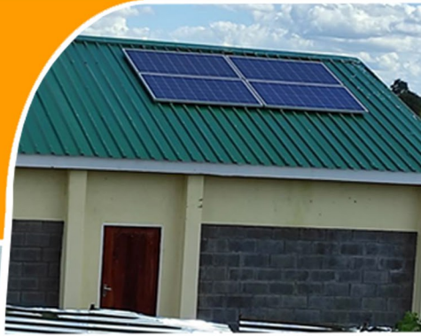
Off-grid Solar System for Village Clinic in Mchinji. 1.1Kw of Solar Inverter and 2.4kwh 24 V Lithium Battery
