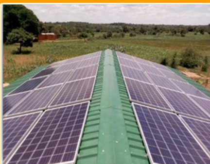
9KWP Three phase solar backup system for cooling milk. Mapuyu Milk Bulking Group- Chileka-Lilongwe
