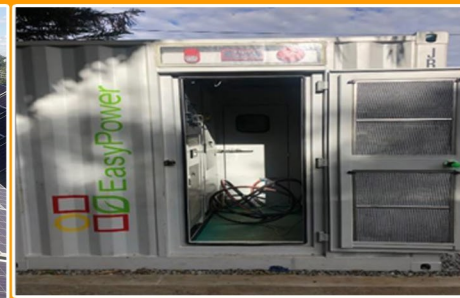
60KWP Hybrid Containerised System for TB Laboratory and offices for Ministry of health at Area 3 Worked with easy power south africa and solarise MW
